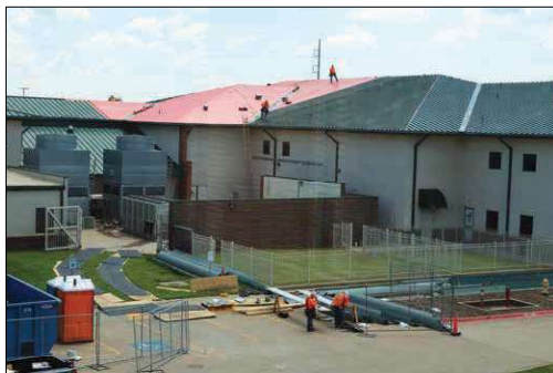
Workers begin making repairs to the Burns Hall roof to repair May 2024 tornado damage.
