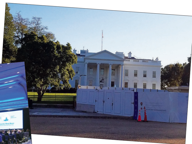
Above photo by Jess Pendergrass The White House hides behind the current renovations that will end in a taller, thicker fence across the front lawn on Nov. 2 in Washington, D.C.. Unlike the current fence, the new fence will obstruct photography of the front of the president's home.
